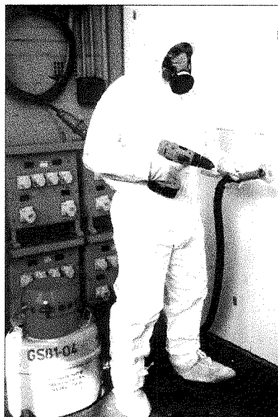
Using a Class H vacuum cleaner and a drill cowl
