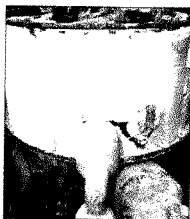
Asbestos lagging on an old tank
